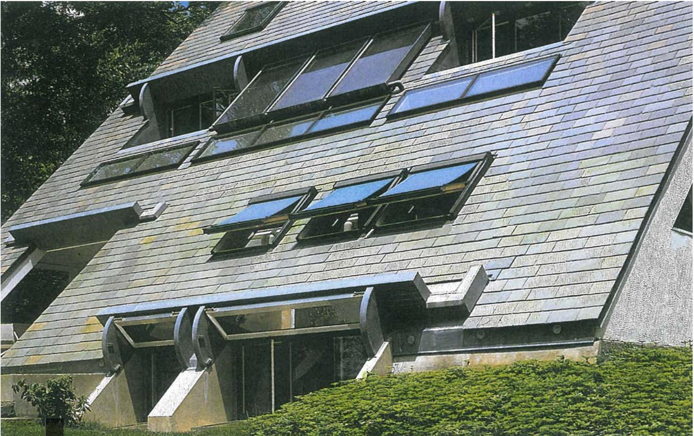
Partial south elevation of the house showing solar heating water panels
