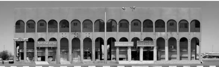
Main bus Station, Abu Dhabi; commercial building in Liwa, western region, Abu Dhabi; residential palace, Al Ain, Abu Dhabi (photos by Marco Sosa)
