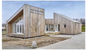
The house is part of the BIOTOPE, which is an exhibition park and resource centre that's designed to showcase the latest in sustainable construction technologies. It is flexible, modular home that can be assembled quickly becasue it is built with innovative digital manufacturing processes. Since the home sits on top of steel piles it can be disassembled and rebuilt in another location, with a different comfiguration.
