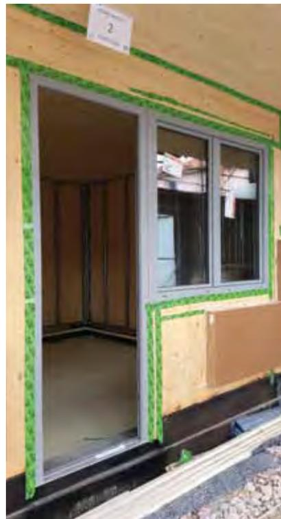
FIG.9 | NASTRATURA DEL SISTEMA DI INFISSI CON ACCOPPIATA FINESTRA E PORTA DI INGRESSO
