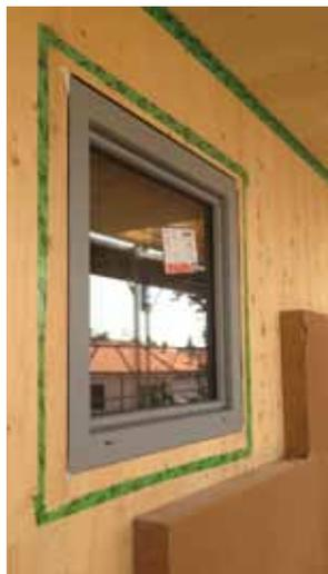
FIG.32 | FINESTRA INSERITA NEL PANNELLO DI CLT SENZA UTILIZZARE IL FALSO TELAIO *SUBFRAME*
