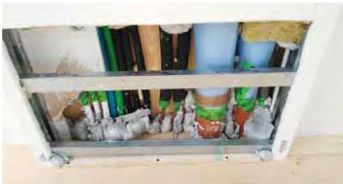
FIG.15 | NASTRI A TENUTA E SCHIUME POLIURETANICHE APPLICATE SUI DIVERSE TIPOLOGIE DI IMPIANTI (LATO INTERNO)
