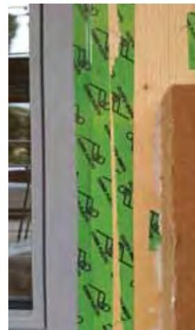
FIG.11 | APPLICAZIONE DEL NASTRO A TENUTA
