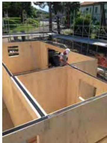
FIG.3 | SIGILLATURA DEI GIUNTI SUL LATO INTERNO CON NASTRO A TENUTA ALL'ARIA
