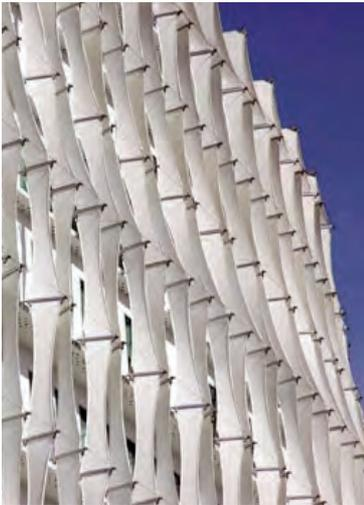
Its use provides and makes powerful the use of natural lighting, allowing it to enter directly and facilitating its diffusion inside the building integrating it with specific elements and systems.
